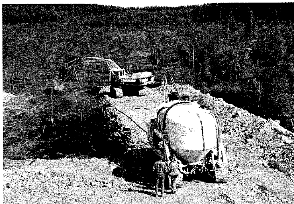
Figur 37 Bindemedel blandas in i delytan
