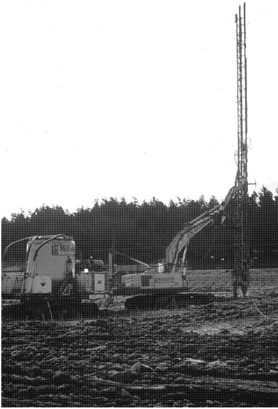
Fig. 8.3 Installation of lime-cement columns at Håby, Sweden.
